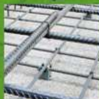
HORMIGÓN ARMADO REINFORCED CONCRETE
